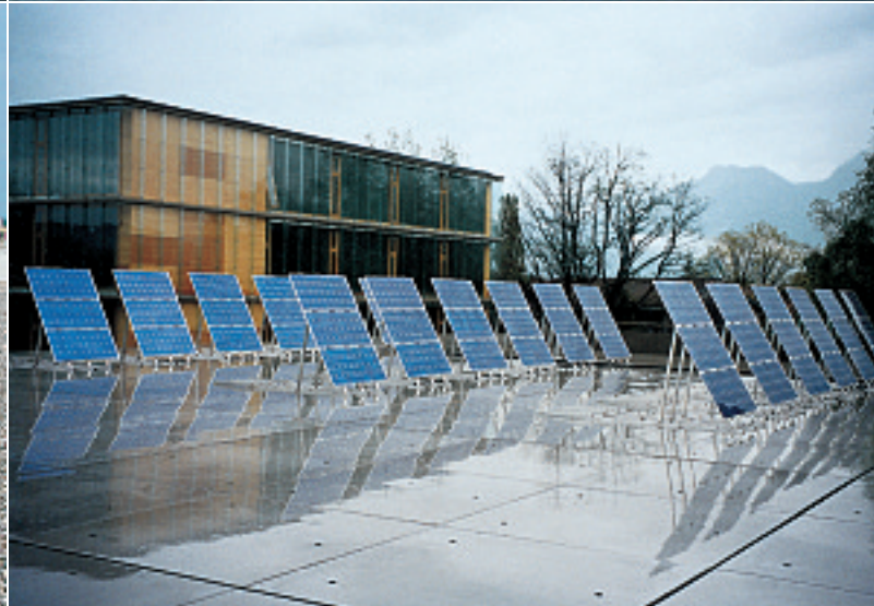
Photos from left to right: KW-Solar, Mahler, Siblik Elektrik, Stromaufwärts
